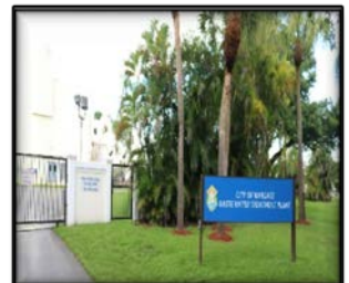
Water and Wastewater Services
